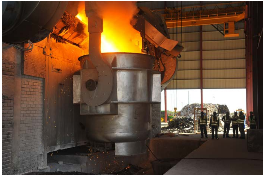
Coega Steels Pty Ltd. (formerly known as Agni Steels SA Pty Ltd.), is the first Steel Melting Unit to have been incorporated in the Industrial History of the Eastern Cape Province, Republic of South Africa. Coega Steels, as it is popularly known, is currently engaged in manufacturing of Mild Steel Billets, using ferrous scrap as raw material
