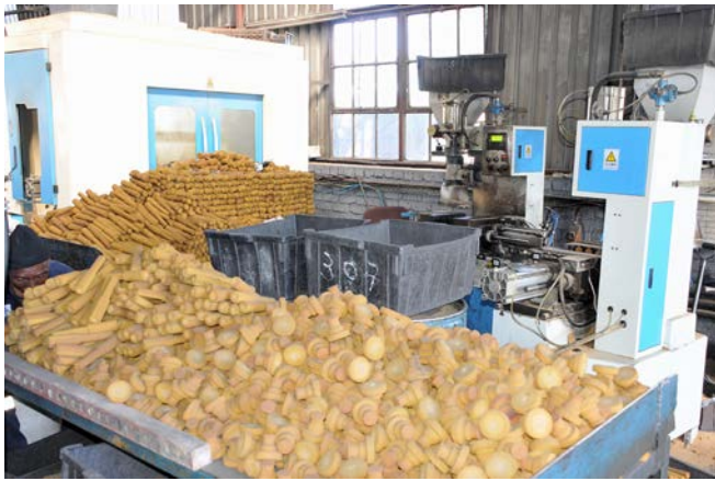
In the coated sand core shooting department, Malleable Castings has two Delin DL361 fully automatic, electrically heated, shell core shooters with a core box size of 400mm x 250mm x 150mm and two smaller units with identical core box capacity
